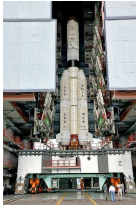
GSLV-F11 integrated up to second stage in the vehicle assembly building
